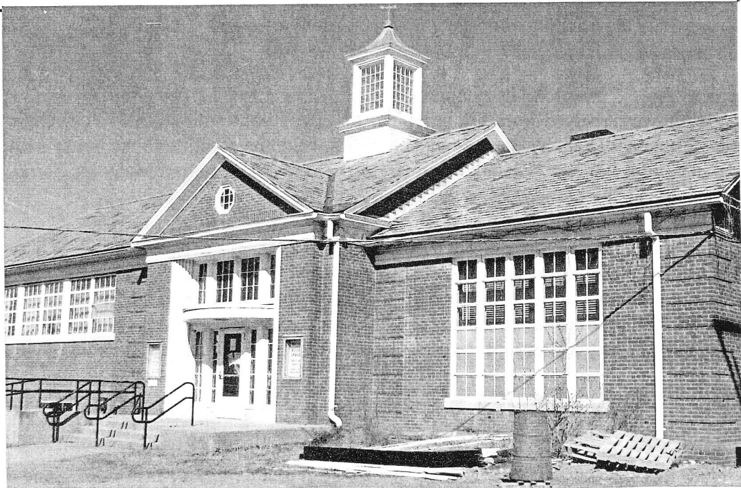
The original Miller Memorial Library, later the Hamden Police Department, demolished 2012.
